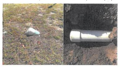
Both above ground and below ground abandonments as seen in these examples are acceptable. Both types of abandonments must be left open for inspection.
